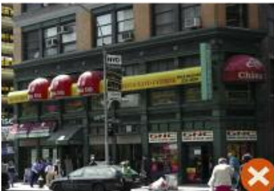
Undesirable - Facade is overcrowded
