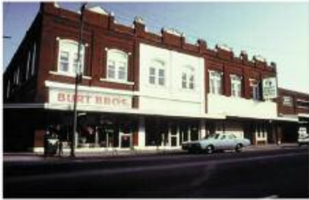
Before - Building façade is broken-up
