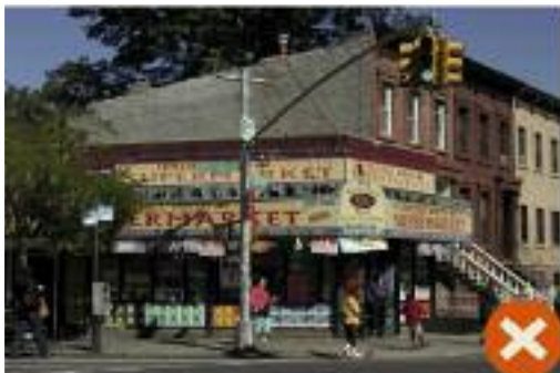
Undesirable - Vinyl awning breaks down under sunlight
