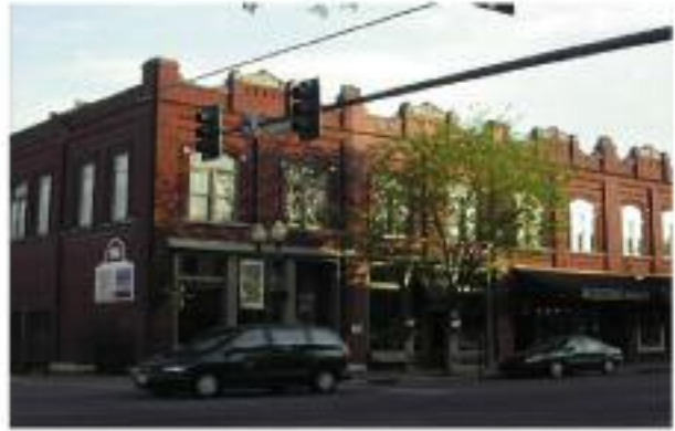
After - Unified façade & signage
