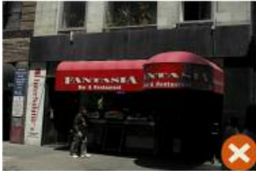
Undesirable - Vinyl awning is too large, excessive coverage
